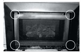
2) Install lower screw below glass door - secure with 4 screws.
